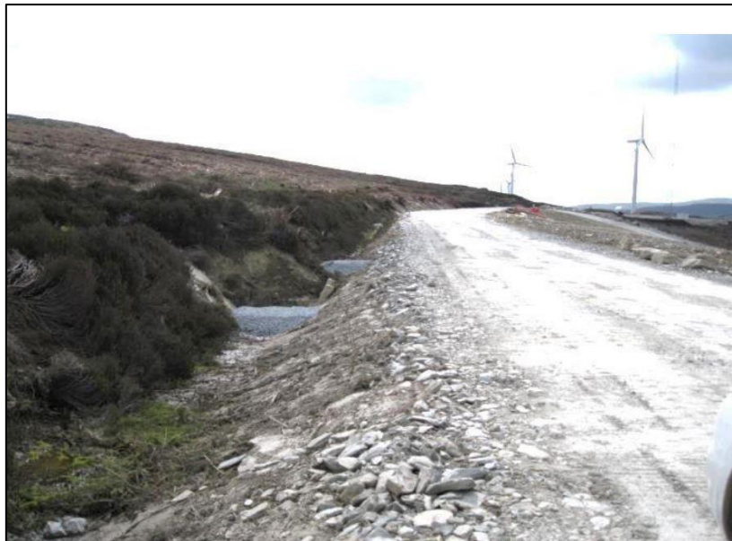
Figure 5-4 Typical example of stones used in a check dam to slow down water flow (Source: SNH, 2015) 5
