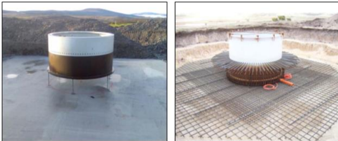
Figure 3-3 Levelled turbine tower can (left) and steel reinforcement being added (right)
