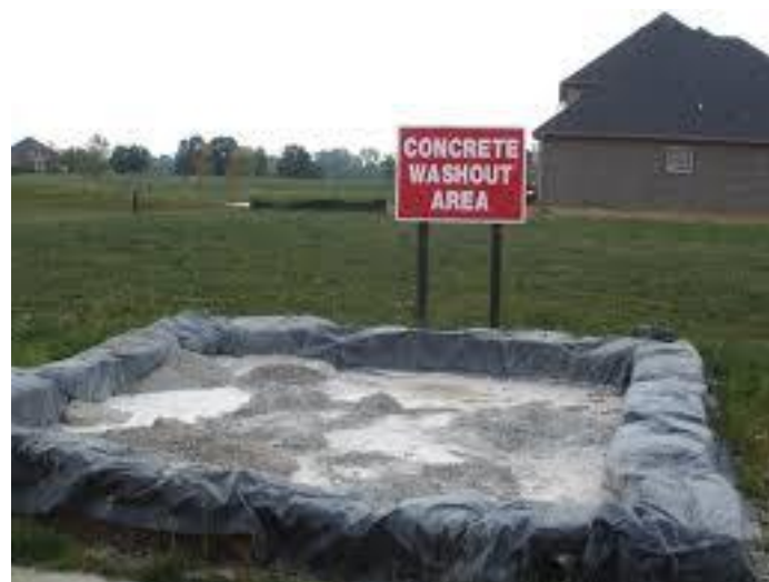
Figure 5-5 Example of temporary concrete washout area
