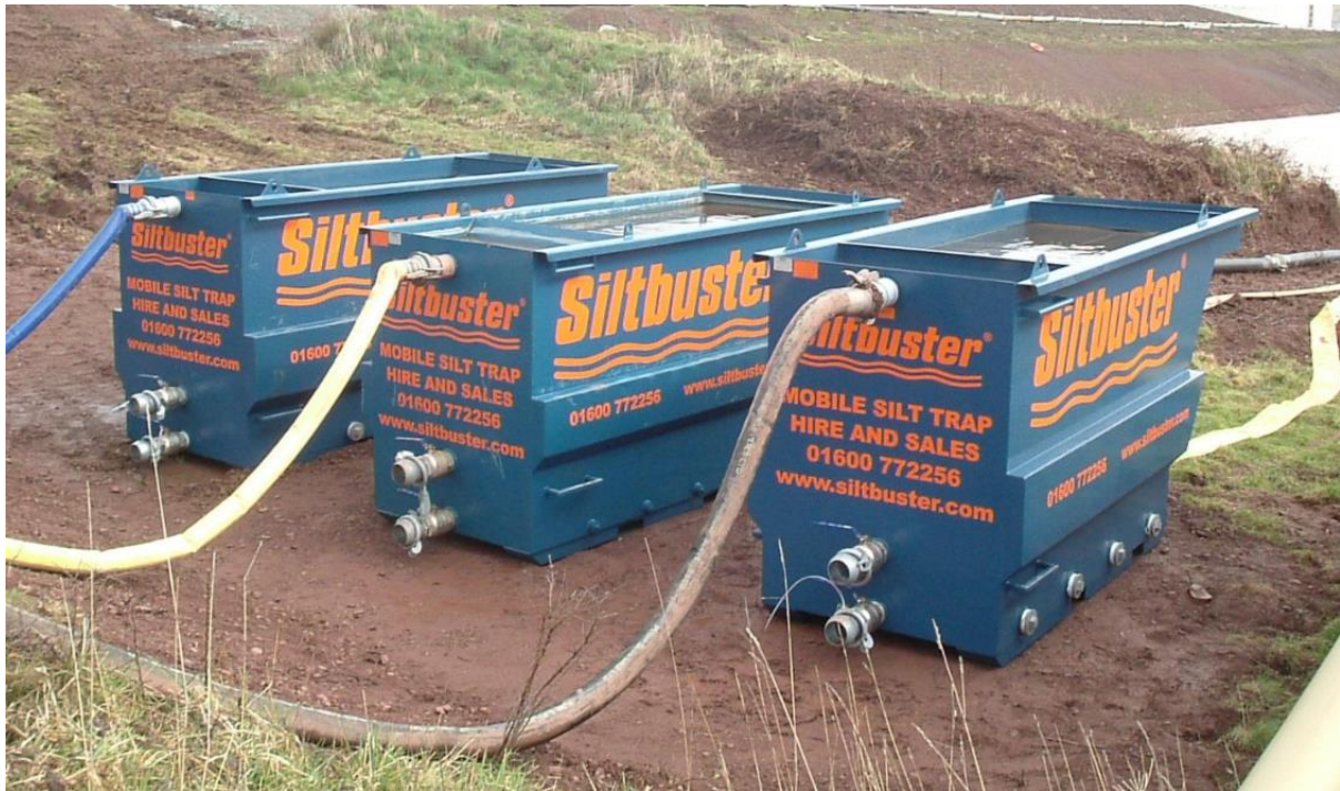
Figure 5-3 Temporary site settlement tanks (Source: Siltbuster)
